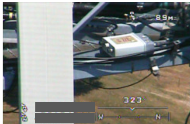
Top Platform Equipment Inspection
